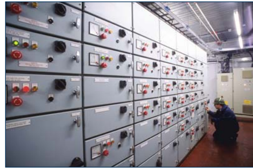
Critical equipment should be protected to prevent data loss and corruption.
